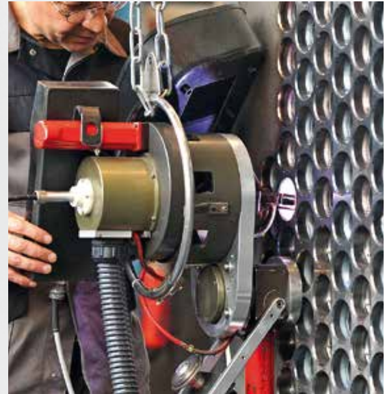
Automatic full penetration tube to tubesheet welding
