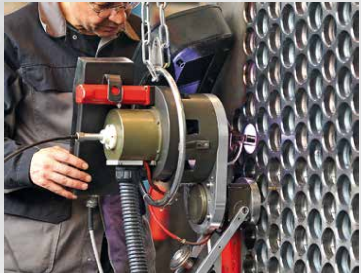
Automatic full penetration tube to tubesheet welding
