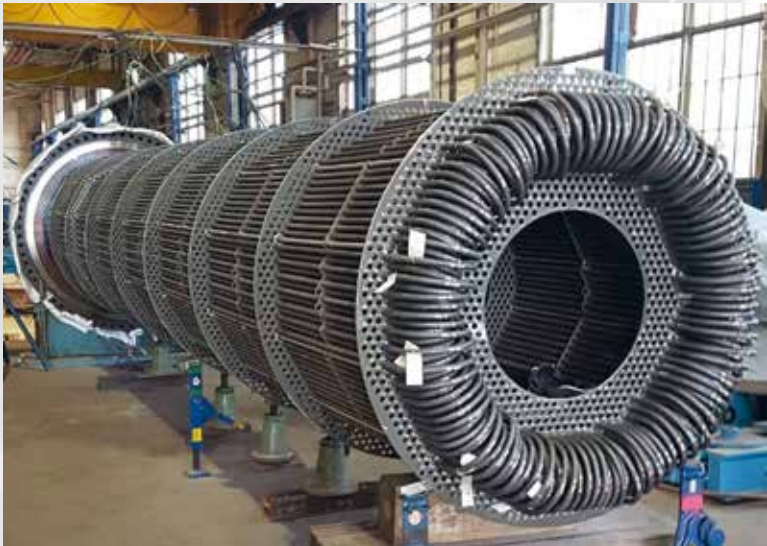
Works construction of a steam superheater
