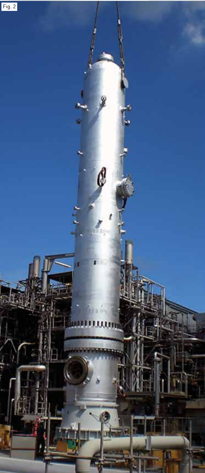
Fig. 1: Synloop WHB on site Fig. 2: Lifting of a synloop WHB on site Fig. 3: Positioning of a synloop WHB on site Fig. 4: Positioning of a synloop WHB on site
